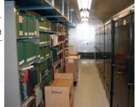
Photo: Joe Arnold, Computer Environments, Livonia, Mich., and Dectron Internationale, Roswell, Ga. | The original prefabricated room envelope that contains the papyrus collection, which consisted of metal skin walls with an excellent R-15 insulation value, was still in mint condition and didn't need updating during the indoor air quality retrofit.
