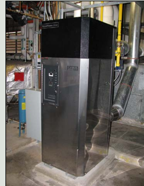
Point of Use High Efficiency Boiler
