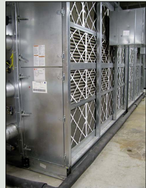
New Air Handler
