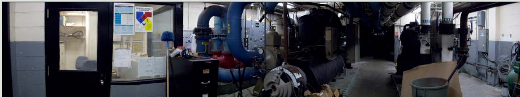
Pre-existing Central Energy Plant
