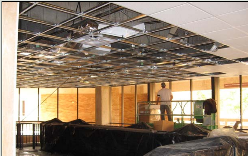
VAV, Controls & Ceiling Upgrade
