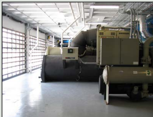
Renovated Central Energy Plant
