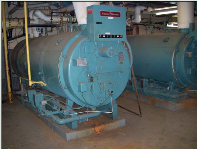
Pre-existing Central Boiler System
